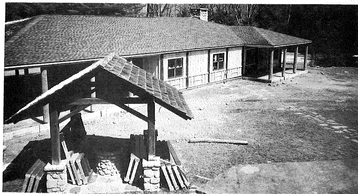
A VIEW FROM THE BUCKLIN PORCH (THE NEW HERITAGE CENTER IS ON THE RIGHT)
